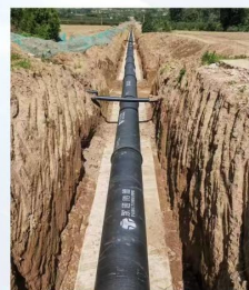
DN1200 pipe for Xiaolangdi Dam diverting water for the Yellow River
