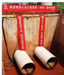
DN1200 Jacking pipe in Jiangxi province
