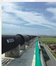
DN1000 self-restrained joint pipe
