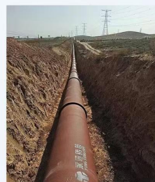
DN600 sewage pipe network for Jiujiang section of the Yangtze river
